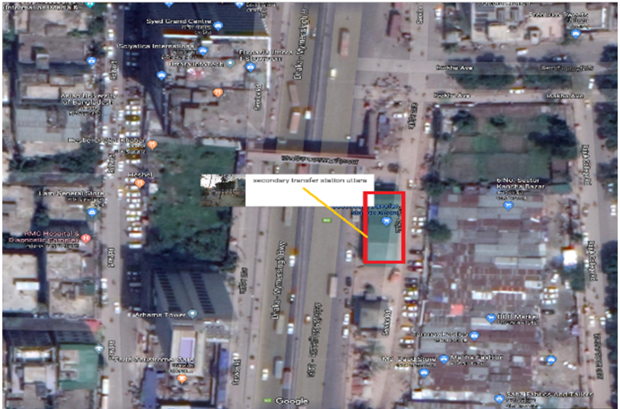
Photograph of Secondary Transfer station, Uttara.
